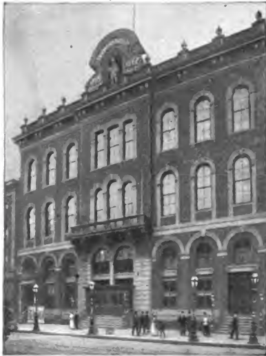
AMMAN HALL, 14TH STREET BETWEEN IRVING PLACE AND THIRD AVENUE.
